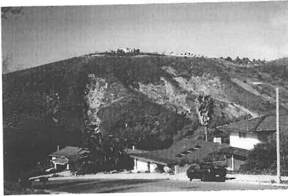
FIGURE 1.11 Urban development The presence of a landslide on this slope suggests that the slope is not stable and further movement may occur in the future. This is a “red flag” for future development in the area. (Edward A. Keller)
