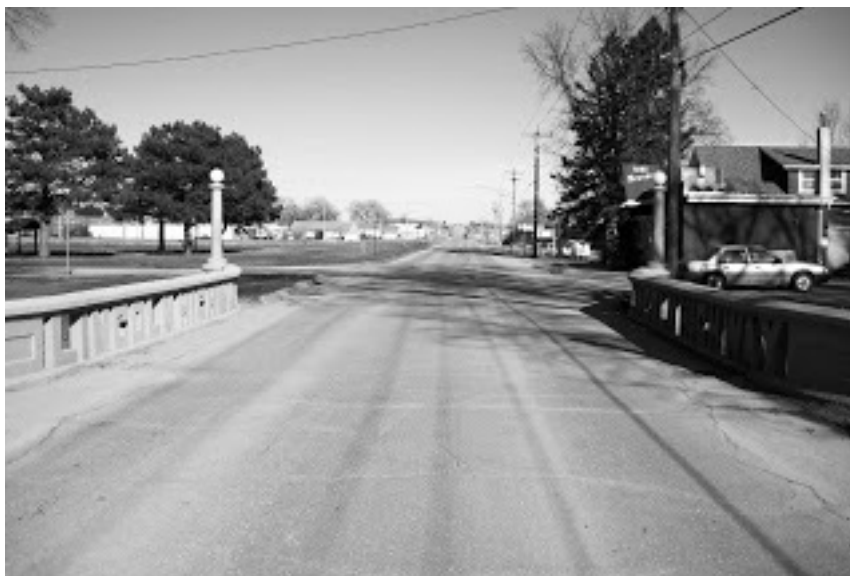
was completed. (Tama: Lincoln Highway Bridge, 2016)
