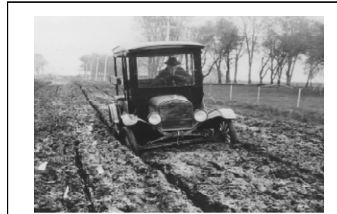
US Hwy 30 during rains before aggregates were used to maintain the roads.
