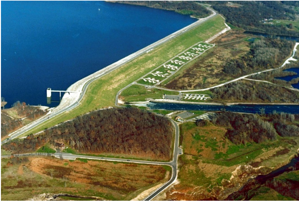
Figure 3. Saylorville Spillway (Wikipedia, Saylorville)
