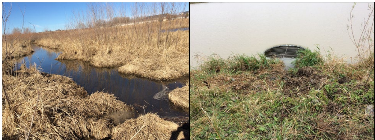
Figure 45. The image on the right is an example of a retention pond constructed in a new housing development in Cedar Falls. Retention ponds can be used to slow the rate of flow and artificially managing water, although the example on the right has a drain where the water would go down into the sewer system instead of flowing naturally into the stream or being infiltrated into the ground. The photograph on the left provides an example of a relatively successful restoration project; Located on UNI's campus, this wetland project is beginning to manage water effectively while providing positive influences on the Dry Run Creek and its overall health.
